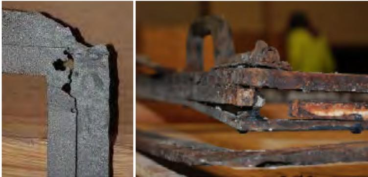
Deteriorated frame from one of the four stained glass windows being restored as part of this phase.
