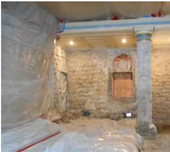
Left, sanctuary wall and column with plaster removed to expose coral construction. High Altar is covered in protective plastic.
